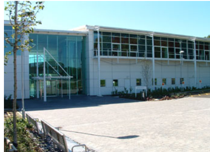
ETL Bangor office at CAST
